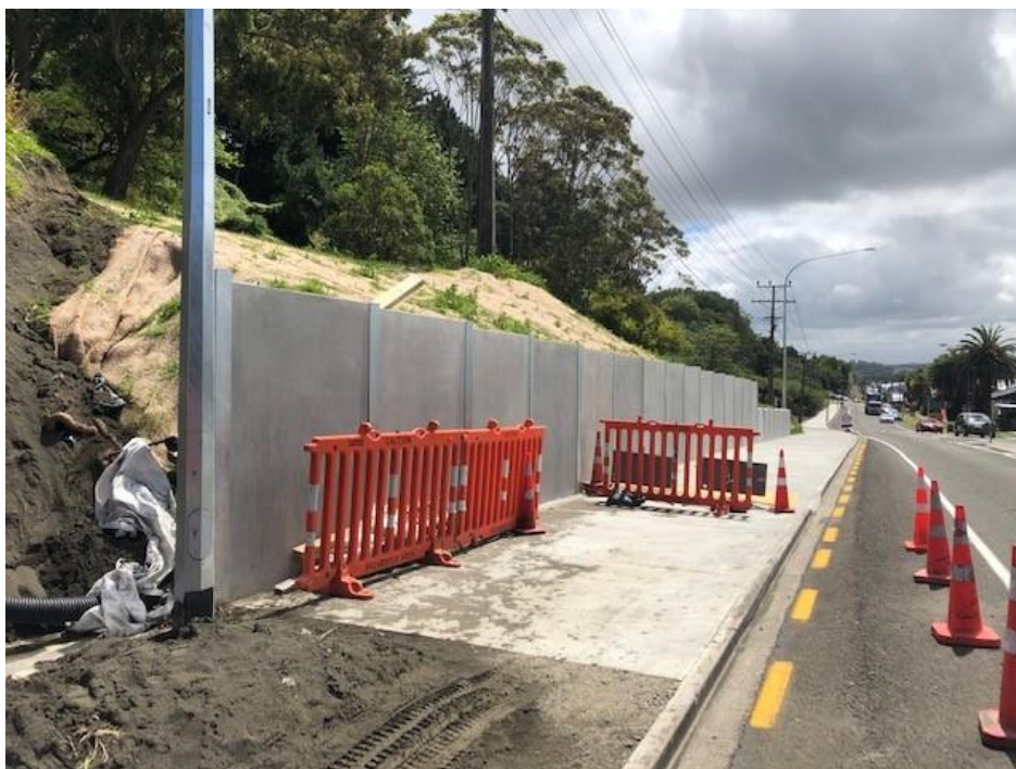
Photo: Retaining tilt slabs in place on London Street Shared Pathway link.
