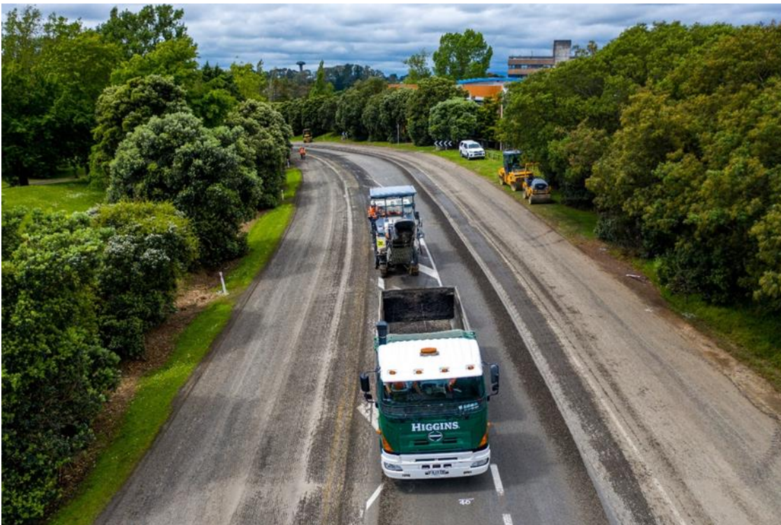
Pavement Sealing Work on Tennant Drive South of Massey University
